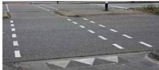
RIGHT: Cyclist lane without priority using only bar markings alongside the lane.
