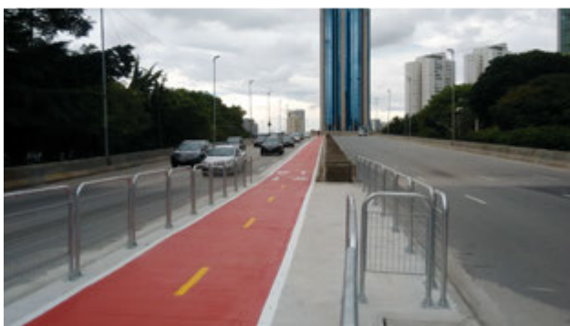
Picture 4 – Photo of the Antarctic viaduct – before and after the intervention (© Google Earth (access on 10/11/2016))
