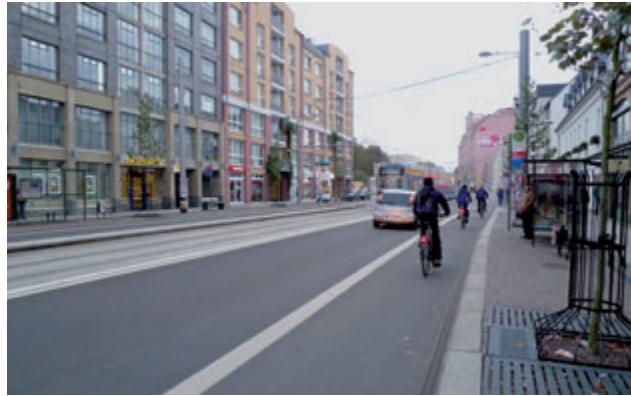
Fig. 2 Re-designed main road, Leipzig (© Jörg-Thiemann Linden)
