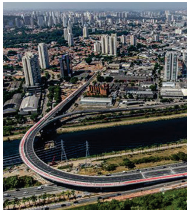
Picture 5 – Aerial photo of Laguna Bridge (© Municipal Communication Secretary)
