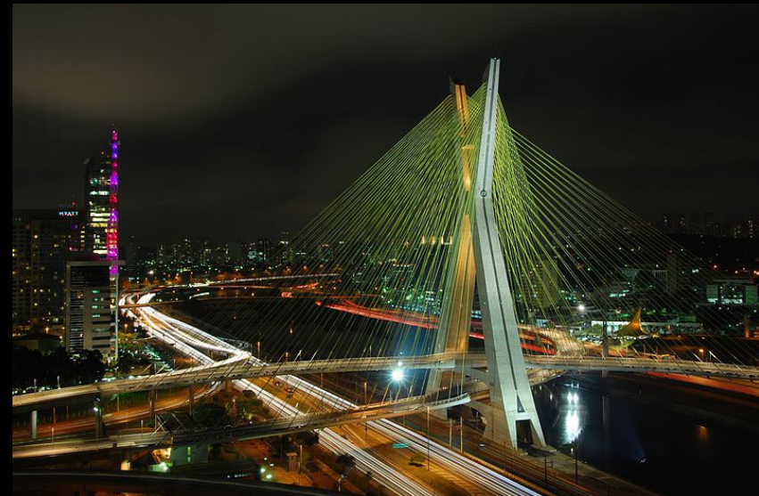
Octavio Frias Bridge, São Paulo
