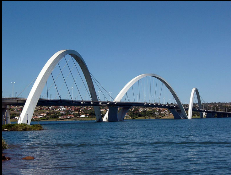
JK Bridge, Brasília
